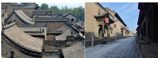
Picture 1 Roof form Picture 2 External streets
